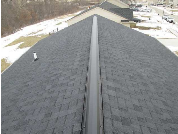
Roof top view
