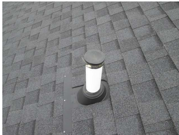
Remove plumbing stack cap
